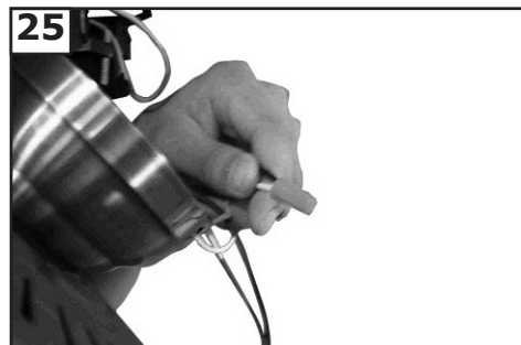
25 Make wire connections to power source using wire nuts provided. Make sure that no filaments are outside of the wirenut. After making the wire connections, the wires should be spread apart with the grounded conductor and the equipment-grounding conductor on one side of the outlet box and ungrounded conductor on the other side of the outlet box.
