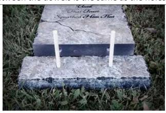
When choosing between rebar and wood dowels, consider the type of soil you have. At our house, we have thick clay and use rebar because the wood dowels simply split apart if we try to hammer them into our dirt.
