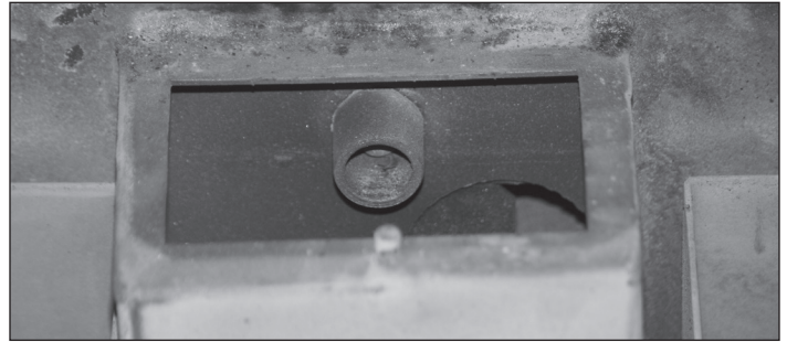
Figure 34: Remove ash from ignitor tube (underneath firepot)
