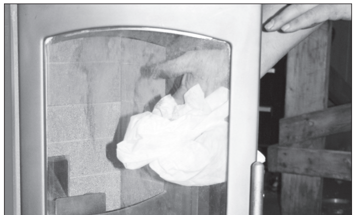
Figure 31: Wipe glass and inspect gasket
