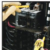
Measure Voltage In Panels
