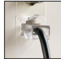
Trace Data Cables
