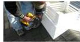
**Step 9:** Position cupola on center of roof and fasten with 3" white headed screws. **Note: if you want to utilize venting, cut a hole (app. 8" square) in the roof prior to fastening cupola. Attach screen mesh over hole to keep bugs out.)**
