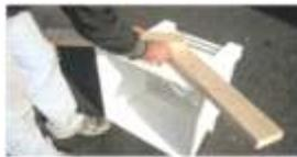
**Step 7:** Use pattern to mark cut lines that match your roof profile. Cut lines should extend from each lower corner to your center line drawn in step 4.
