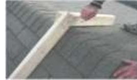
**Step 3:** Lay your boards over the peak of the roof, making sure each board is fully against the surface. Mark boards with pencil to confirm angle position. Mark front & back of roof (not all roofs are symmetrical.)
