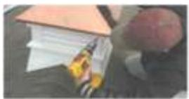
**Step 11:** Attach roof to base using 1-3/4 in. white headed screws supplied with unit.
