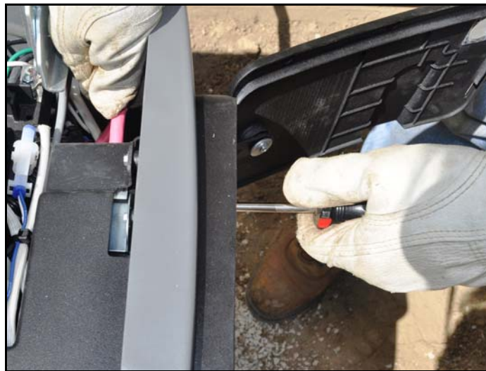
Figure 6-2. Câblage c.a. principal
