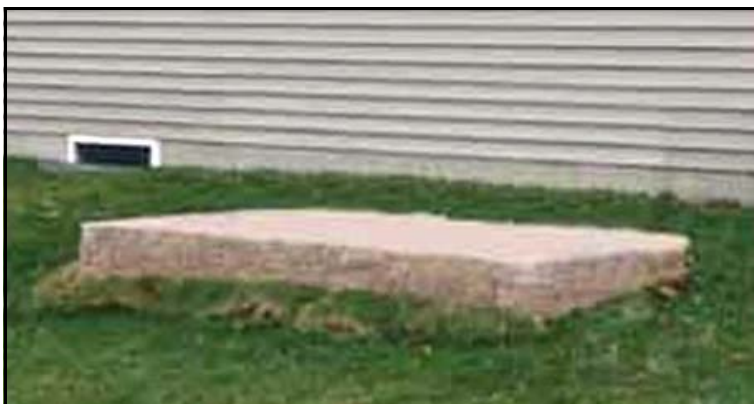
Figure 3-4. Concrete Pad Site
