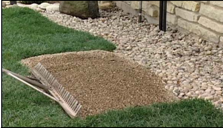
Figure 3-3. Compacted Gravel Site
