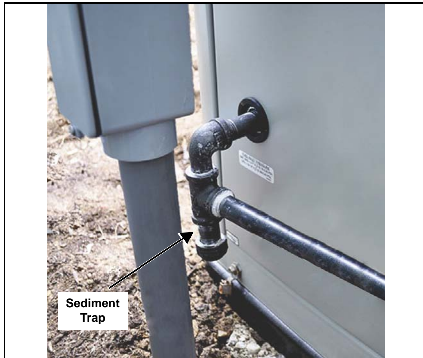
Figure 5-3. Sediment Trap
