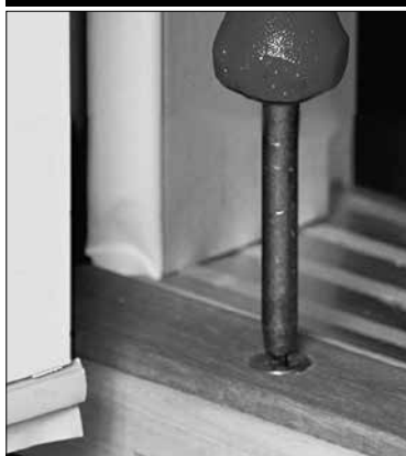
FIGURE 28: Raise or lower the sill by adjusting the sill screws. Some sills may have covers over the adjusting screws. These covers must be removed prior to making any adjustments.
