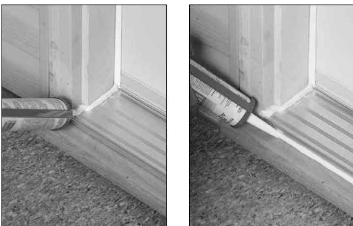
FIGURES 24 and 25: Caulk the sill crown and the front of the sill.
