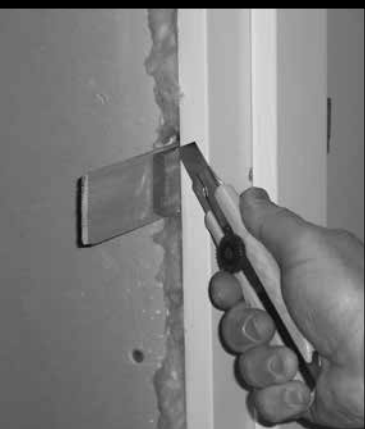
FIGURE 23: Insulate between the jambs and the wall studs all around the door.
