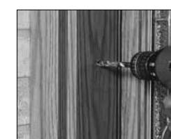
FIGURE 20: Pre-finished systems must have holes drilled before screws are installed.
