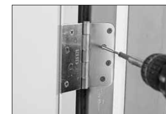
FIGURE 19: Install 2-1/2" screws through the lock jamb into the shim and stud. Minimum of 3 locations
