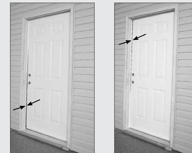
Figures 8 and 9: The weather-stripping on these doors is not evenly compressed.
