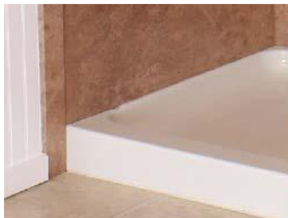
Vertical trims installed outside shower base
