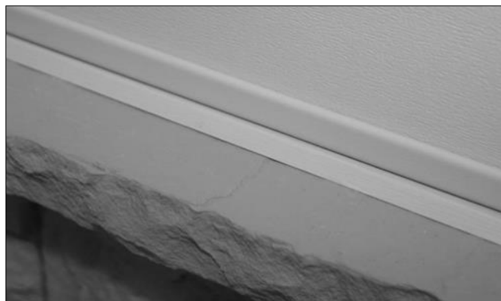
Flashing Covering the Screw Heads
