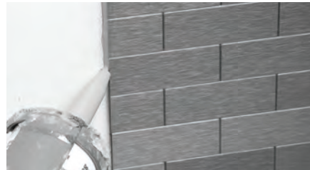
Finishing option 2: Caulking outside edges
