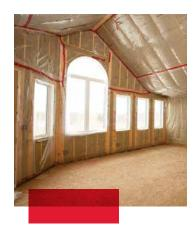
ROCKWOOL COMFORTBATT® is a semi-rigid batt insulation designed specifically for exterior wood and steel stud applications in residential and commercial construction. Made from natural stone and recycled slag, ROCKWOOL stone wool is a high-density insulation that will fit snugly into wall cavities and will not slump over time. It also adds superior acoustical performance to wall assemblies and floors and can be used in acoustic applications required by building code.
