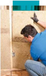
ROCKWOOL cuts quickly and accurately with a serrated knife, such as a bread knife, so you can easily achieve optimal fit around pipes, electrical boxes, wiring, ductwork and between studs and joists that are less than a standard width.
