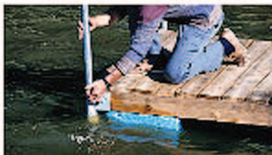
Lower pipes to lake bottom
