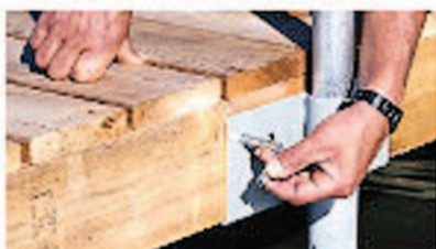
Use L pin to lock sections
