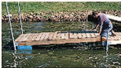
Float dock into position
