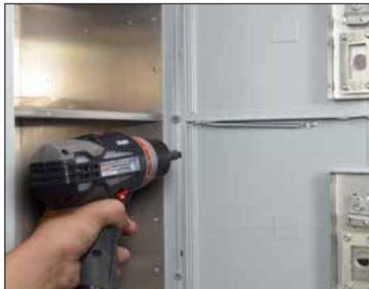
Figure 5D – Secure units together using connector machine screws
