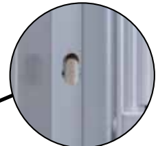
Connector kit mounting hole
