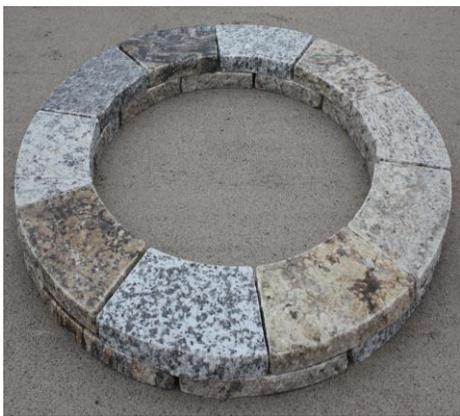
**Step 3:** Install second row of granite blocks (10 units). Place the first block on top of the bottom block staggering the intersection of two blocks on the row below. Continue around the circle making slight adjustments as needed so that the edge of the blocks fit tightly in the circle. Remove one block at a time from the second course and glue to the two blocks below using quarter-sized dabs of concrete adhesive.
