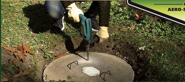
Drill 5/8" hole for airline to exit septic tank
