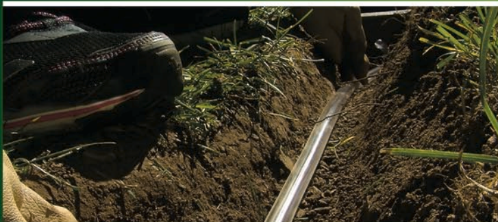
Dig trench and bury airline 2" - 3" underground
