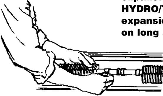
All piping expands when heated. In shorter runs, the movement of the risers in their holes will take care of expansion. But on longer runs, it's wise to install an expansion compensator to prevent strains at the joints and buckling of the elements. Install a Hydro/Tite at the center of a long run.
