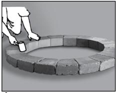
**4.** Place 19 wall block units on top of paver base. Lay them tightly together to form the circle. Level each stone front-to-back and side-to-side. Make sure each stone is even with the previously leveled block. Use a rubber mallet to level.
