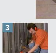
Attach floor runner using concrete
