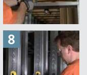
Snap in grommets for electric and plumbing.
