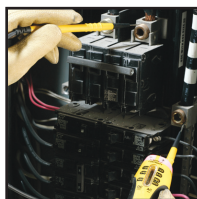
Measure Voltage In Panels
