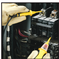
Measure Voltage In Panels
