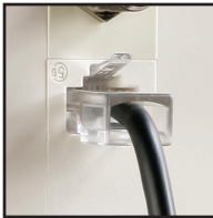
Trace Data Cables
