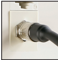
Trace Coax Cable
