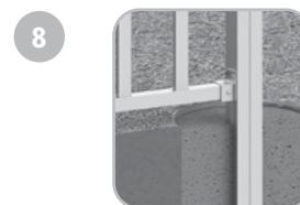
Level and brace the second post. Mix and pour the concrete into the second hole.
