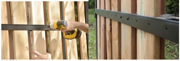
ALWAYS screw in both top and bottom screws in each fence-board before fastening the next fence board. following this instruction will eliminate any sag in the stringer.
