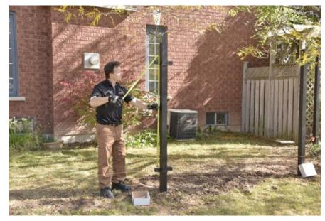
It is at this point that if you are running a string line to follow the grade instead of stepping your fence, that you should measure approximately 12" up from the ground to the bottom of your bottom End bracket collar and hand tighten the bottom bracket.
