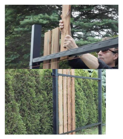
If following the grade, make sure that the fence board tops are the same distance from the stringer all the way along the fence section for a nice even looking fence project.
