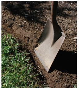
Score the ground along the desired layout creating a vertical wedge at the desired depth.
