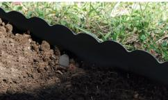
Backfill edging continuously to ensure straight lines, compacting both sides.
