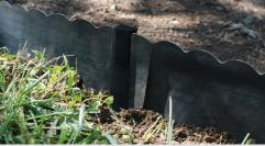
Insert edging and hammer anchoring stakes (included) along installation. For typical installations use a suggested minimum of one stake every 4'. Additional stakes available and sold separately.
