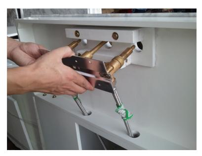
**Step 4:** Screw in wood screws through the back of the mounting plate into the spacers. You are now completed with the off-the-wall wall-mount system (installation time about 10 min.). Follow the instruction for the faucet trim to complete the faucet installation.
