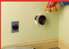
H Dryer Vent
