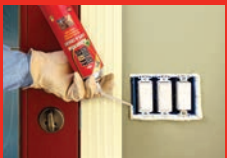
C Electrical Outlets
