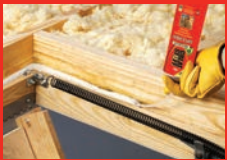
A Attic Hatch
