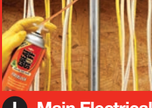
I Main Electrical Panel
