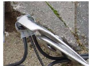
10. Repeat steps 8 & 9 using the smooth sides of the power supply cable and the other wire from the light. You should end up with two connections per light as shown. **After all lights have been attached, plug in and switch on the transformer to test all connections.**
