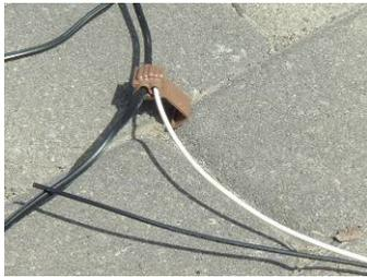
11. Connectors should be buried below the pavers in the sand setting bed, in the ground, or in the stone behind retaining and garden walls.
