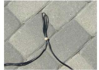
7. When using the silicone connectors cut the power supply cable in half where lights will be located and split it down the middle. Note that one side of the cable is ribbed and one is smooth. Do not strip the insulation from the cable. See back of sheet when using the brown connectors.
