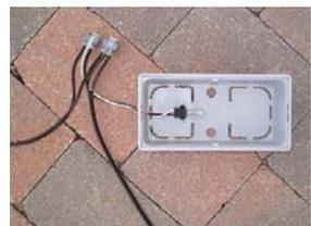
Note: When you reach the last light on the string, you will only use two holes on each connector as shown.
