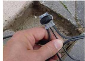
9. Once you have all three wires in each of the three holes and pushed all the way to the back, squeeze the connector with a pair of pliers to push the black cap down. This will make the connection between all three wires and will require some force. The connectors also contain silicone to protect the connection from moisture which may squeeze out on this step; be careful not to get it on your clothing.
