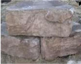
**Step 3:** Install second row of blocks (12 units). Place the first block on top of the bottom block staggering the intersection of two blocks on the row below. Continue around the circle making slight adjustments as needed so that the edge of the blocks fit tightly in the circle.
