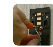
The wiring must be connected to a transformer with a voltage of 8VAC - 24VAC and an internal
