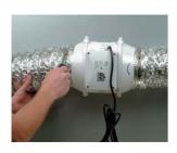
Attach the ducts with clamps.
