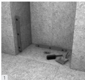
**GB** Cut the 2" pipe flush to the surface of the floor construction. Make sure that the cut out fits to the One Step base drain. Cut out a 5" diameter hole around the 2" pipe to allow the wedi drain to be inserted into the subfloor. The drain and trap have to be sturdily fastened to the sub floor.
