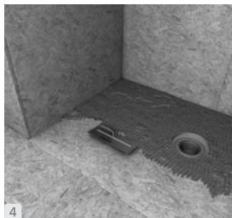
**GB** Apply a bed of modified thinset on the floor using a minimum 3/8" x 3/8" or max. 1/2" x 1/2" square notch trowel. The whole contact area for the base must be covered.
