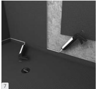
**GB** You can now install water-proof wedi 1/2" building panels directly to the framework and seal all joints and fastener points as usual and per wedi building panel installation guidelines. (you may install other Backerboards but have to add topical waterproofing/membranes).
