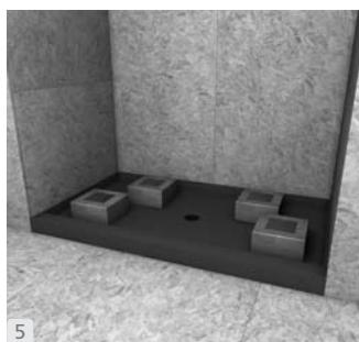
**GB** Press the Fundo One Step firmly into the thinset bed, ensuring that the installation is level and void free. Apply some weight equally and for at least 30 minutes (thinset bags).
