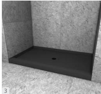
**GB** Dry fit the base and make sure that floor drain is located in the center of the wedi drain. Make sure the base walls are square and tight with the framework.
