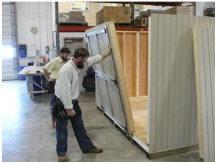
Continue installing panels per diagram
