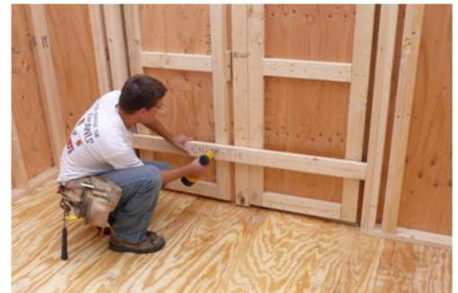
On the inside of the doors you will find a 2x4 brace. Remove the brace and set aside, you will use it again to help brace.
