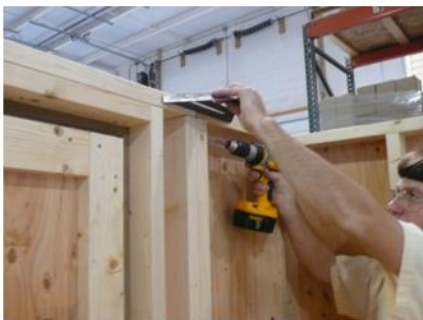
Use angle and make sure 2x4's are flush, and secure with 2 1/2" screws.
