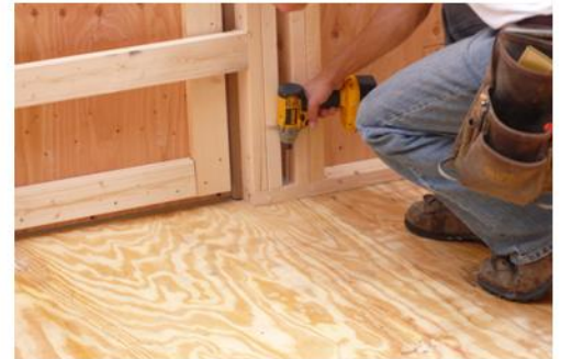
To completely secure, fasten with 2 1/2" screws into 2x4 through the floor.
