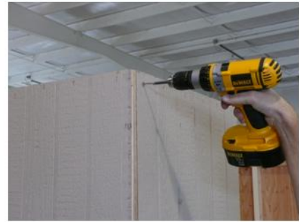
Fasten outside wall corners with 1 1/4" screw to hold wall in place.
