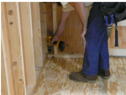
Secure wall with 2 1/2" screw.
