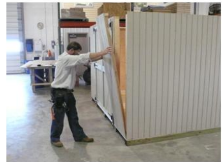
Continue installing panels per diagram.
