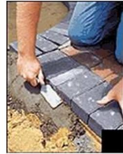
🗨 In southern climates not subject to freeze thaw, a concrete toe can be added instead of using edge restraints. This is not recommended for driveways in any climate.
