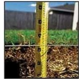
🔍 Measure the depth of your excavation frequently. Measure from the line, not from the surface of the ground.
