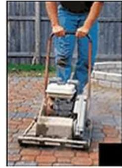
Use the plate compactor to set the pavers in place.
