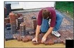
🔍 Lay the pavers working out from one corner. Keep your lines straight, and work from on top of the pavers you have already installed.
