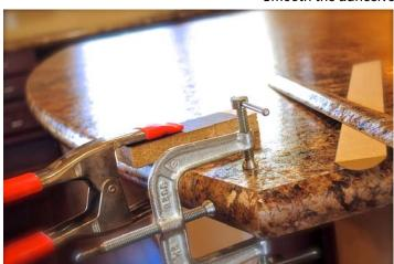
substrate. Use fiber-reinforced tape applied every two to three inches down the length of the molding and around the corners vertically to secure miter corners. (**FABTIPS:** Use a laminate faced wood block and 3" pinch clamp to maintain correct height of molding to the laminate countertop edge—see photo at left).
