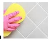
Haze may also be removed using a damp clean terry cloth or cotton towels Remove haze by dragging the damp cloth flat over the surface. A final rinse may be necessary if haze is present after 24 hours
