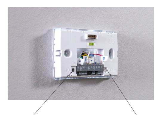
Back glow switch Switching this "On" illuminates the thermostat base. Make sure you switch this to "Off" after installation so you can still operate this feature from the thermostat display.
