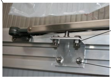
opener with self-tapping screw pan head 4,2 x 13 (S9) screw
