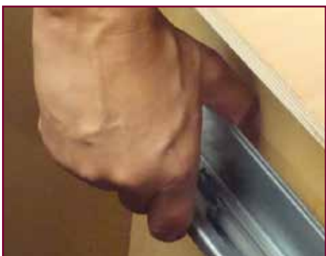
3. Firmly grasp runners at rear of cabinet and slide toward center of cabinet.
