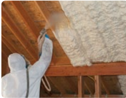
Spray Foam Insulation
