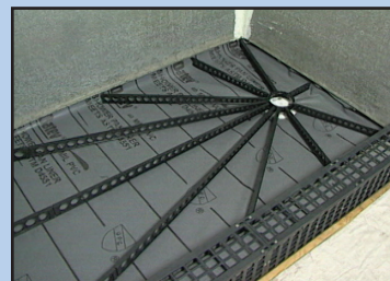
Quick-Pitch® Standard and Extended and Kirb-Perfect® installed.
