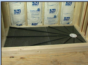
Pre-Pitch™ Standard and Extended installed in rough-in.
