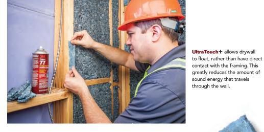
**UltraTouch+** has a Class-A Fire Rating and provides R13 Thermal performance
