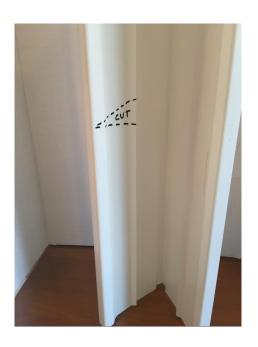
Step 4: Grab the lip of the other Clip-On SuperCorner<sup>™</sup> fold and lift it over the edge of the opposite J Channel until it snaps into place. Repeat over and over until the both sides of the Clip-On SuperCorner <sup>™</sup> is fit tightly onto the the smaller vinyl corner.
