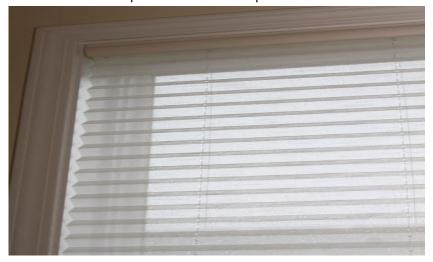
2. Measure from the top of the inside of the window frame to the bottom of the windowsill.
