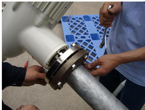
② Connect the turbine to the pole by bolts.
