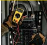
Test Circuit Breaker Panels
