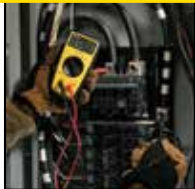
Test Circuit Breaker Panels
