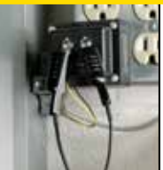
Test AC/DC Voltage
