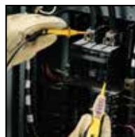
Measure Voltage in Panels
