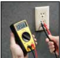
Measure Voltage at Outlets
