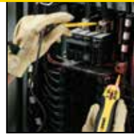
Measure Voltage in Panels
