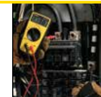
Test Circuit Breaker Panels
