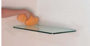
STEP 6 – PUSH THE SHELF IN PLACE. THEN USING A WET SPONGE CLEAN ALL EXCESS CAULKING. LET IT DRY OVER NIGHT. IF NECESSARY, YOU MAY PATCH AND PAINT ANY GAPS FOR A BETTER APPEARANCE.
