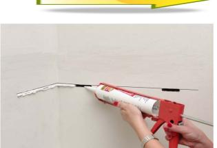
**STEP 5** – APPLY 3/8" BEAD OF CAULKING ADHESIVE JUST BELOW THE LINES, AND IN THE GROOVES. INSTALL THE SHELF IMMEDIATELY BEFORE THE CAULKING DRIES .AFTER INSTALLATION, FILL ALL GAPS WITH MORE CAULKING IF NEEDED.
