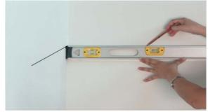
STEP 2 – USE A LEVEL AND DRAW TWO LEVELED LINES AT ABOUT THE SAME LENGTH OF THE SHELF, ONE AT EACH SIDE OF THE WALL WHERE THE SHELF IS GOING TO BE INSTALLED.
