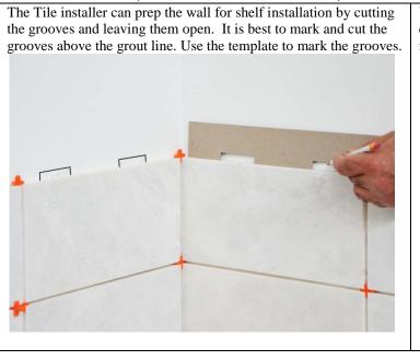
You may have to cut the tile backer board to let the shelf in. Shelf can easily be installed after the grout is done and dry. Follow instructions in step 5 & 6 to finish the installation.
