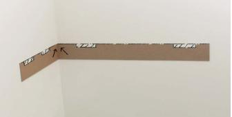
**STEP 3** – USING THE SUPPLIED TEMPLATE MARK THE POSITION OF THE GROOVES ON THE WALL. THE ARROW ON THE TEMPLATE MUST POINT TO THE CORNER.
