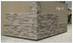
**Note:** There are 4 patterns of the Ledgestone Outside Corner. 2 Left patterns and 2 right patterns. Check for numbers on the backside of the piece. They are numbered 1 through 4. Alternate left and
