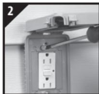
**2** Align keyholes on base with screws and slide to the left. Tighten screws until snug (avoid overtightening).
