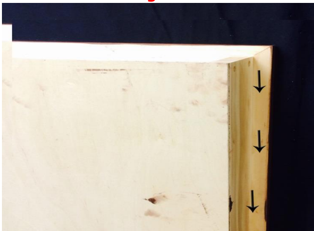
Image 3 Apply Construction Adhesive Around the Edge of the Cabinet.
