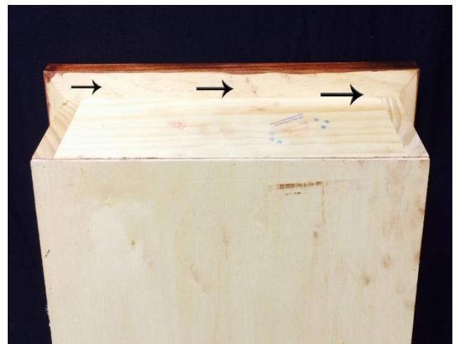
Image 4 Apply Construction Adhesive
