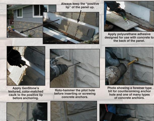
hole and one of many types of concrete anchors.
