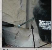
Drive concrete anchor to a depth of 1/8" below flush.
