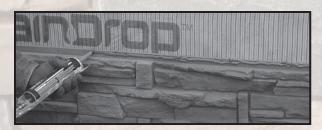
Apply a <sup>1</sup>/<sub>4</sub>" bead of GenStone color matched caulking or polyurethane construction adhesive to all positive edges to ensure a water-tight barrier. This positive shiplap edge should always be upright.
