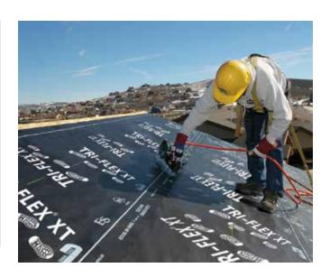
Suitable for use under all major roof coverings - Tri-Flex® XT mechanically-attached underlayment can be used under shingles, tiles, slate, metal and cedar shakes. Refer to subsequent sections for more details.
